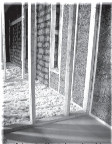
High levels of insulation and careful attention to airtightness on a building designed and partly built by Chris Morgan for his mother whilst working at Gaia Architects. All the materials used are natural and non-toxic; the floor and roof insulation are of sheepswool, and the timber framed walls are infilled with woodchips and straw mixed with clay. The walls are rendered with clay inside and out. Design: Gaia Architects
