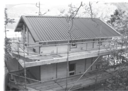
A simple, symmetrical, steel-profiled roof with no dormers or rooflights on a North Woods house under construction this year in the Highlands - installed in two days.
